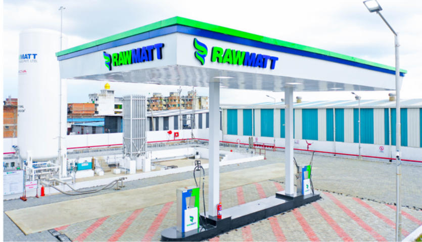
L-CNG STATION IN NAGPUR
